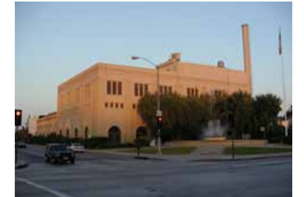
Glenarm Power Plant
