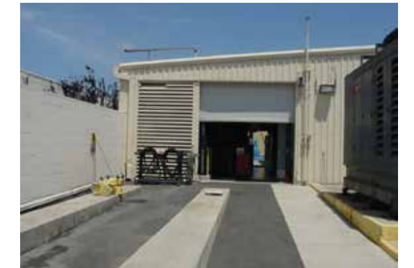
Anaheim Memorial Central Plant Upgrade
